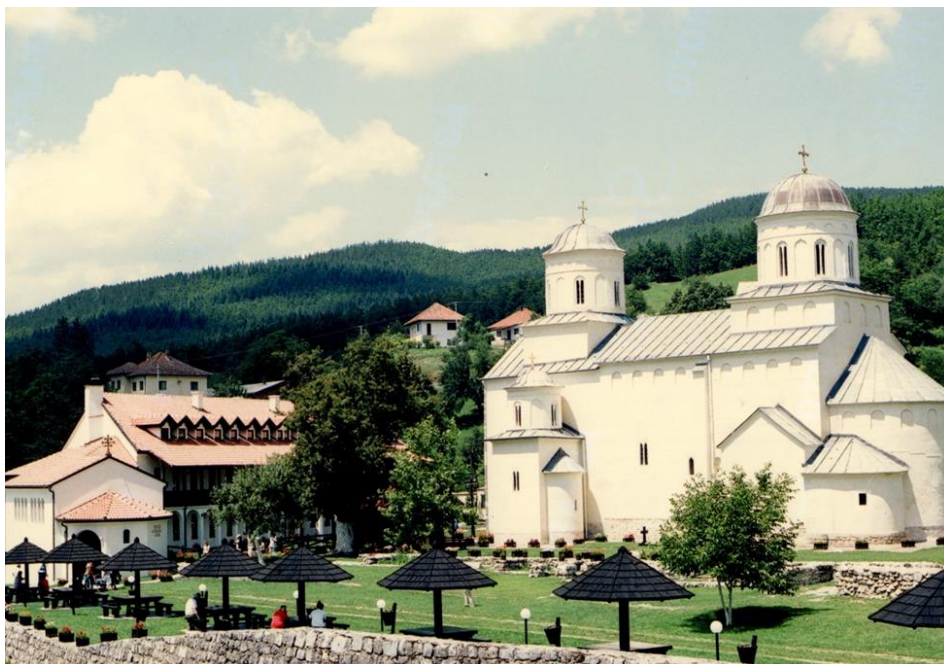
Fig. 2. The monastery complex of Mileševa is protected by law
