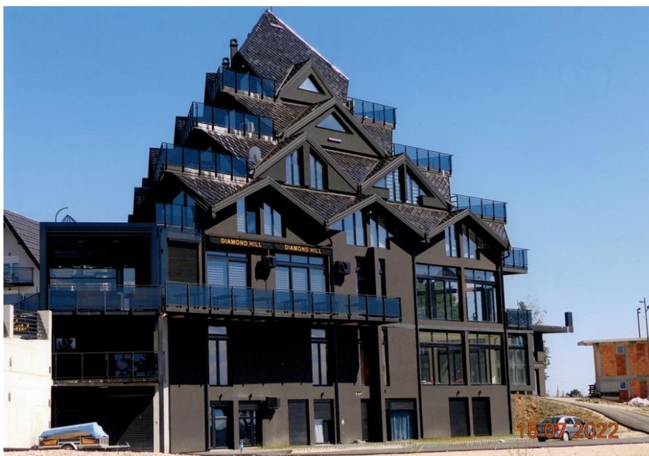
Fig. 3. The Diamond Hill facility in Divčibare
