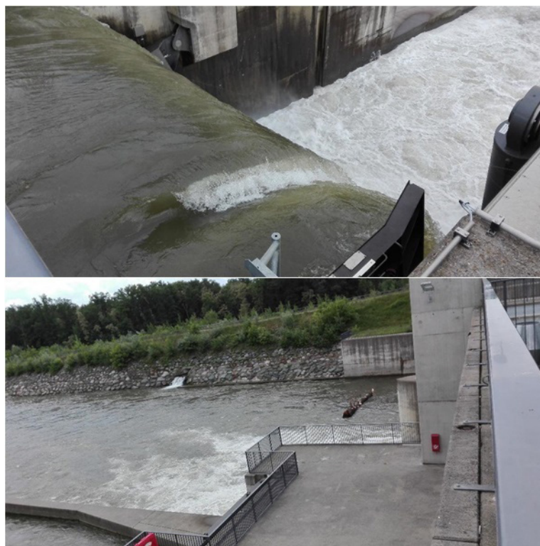
Figure 4. Hydropower plant on the Mur River (Regional park Murauen) (Source: authors)
