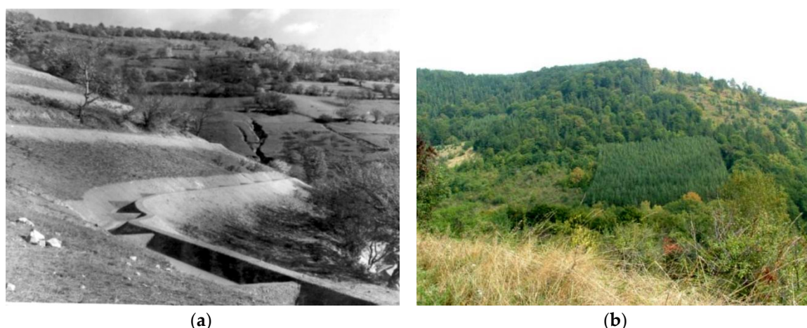
Figure 3. Contour ditches and afforestation of bare land: (a) 1953 [58]; (b) 2016 (photo: S. Braunović).
