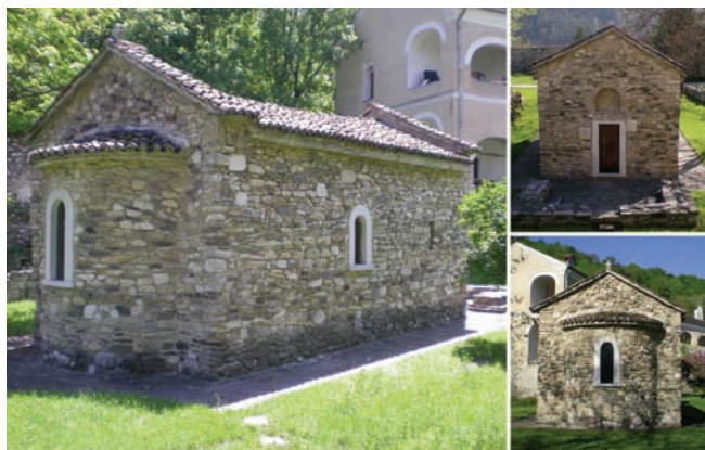
Figure 2. St Nicholas' church: views from the northeast (left), from the west-northwest (right, above) and from the east-northeast (right, down)
