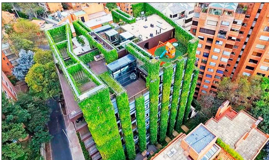
Figure 6. Building Santalaia in Bogota, Colombia (inhabitat.com)
